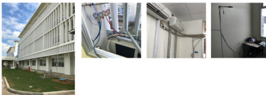
Fig. 1. Installation of the Open-loop GSCS.
